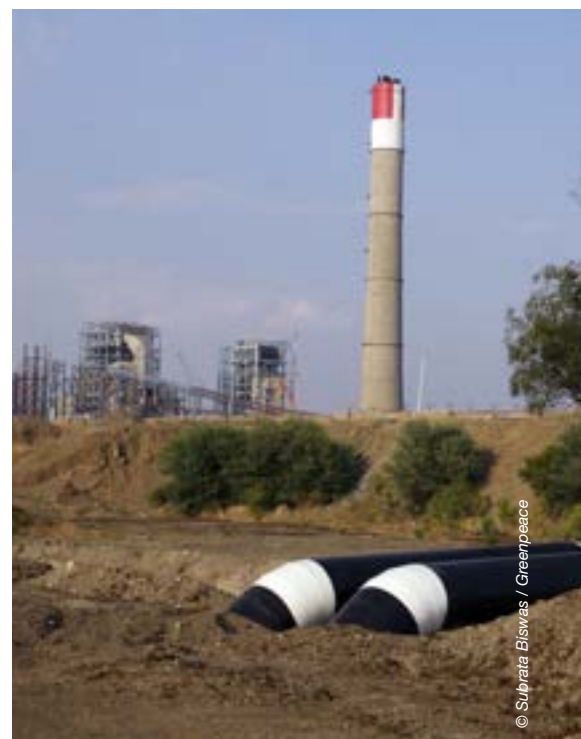
NTPC's Solapur power plant under construction, 2016.
