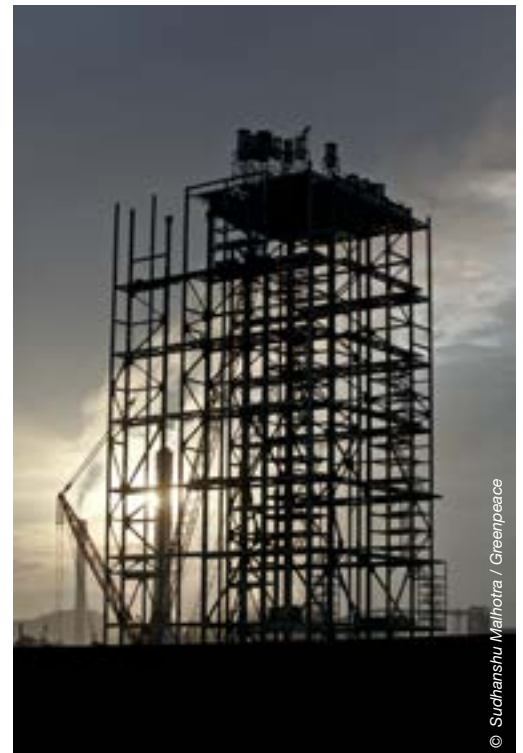
"Anpara-D", a wing of the Anpara thermal power plant, 2011.
